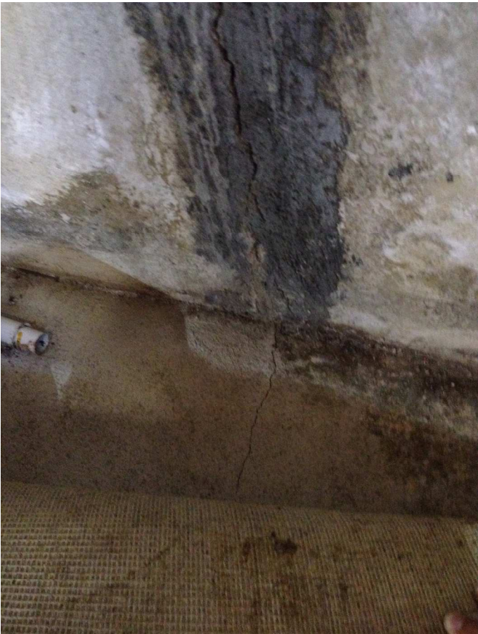
Interior of crack shows floor involvement
