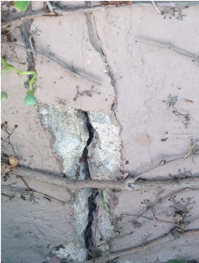
Driveway side - crack at foundation - it has seen previous repair and reopened
