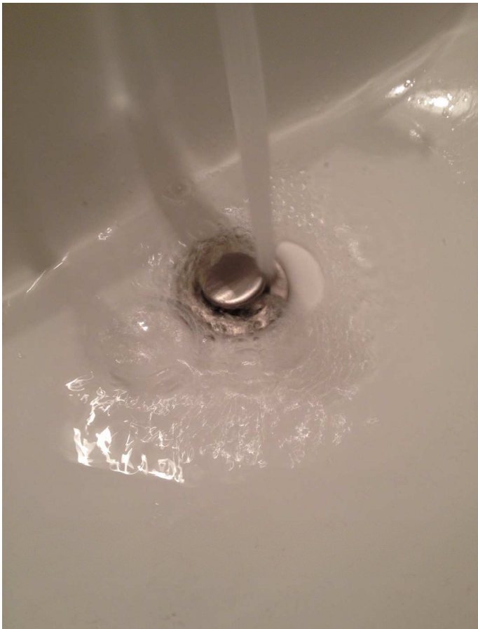
popping sound here and whine in upper toilet may be due to poor venting.
