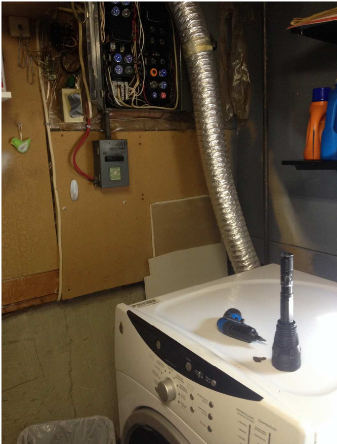
1 meter clearance in from of panel is code
