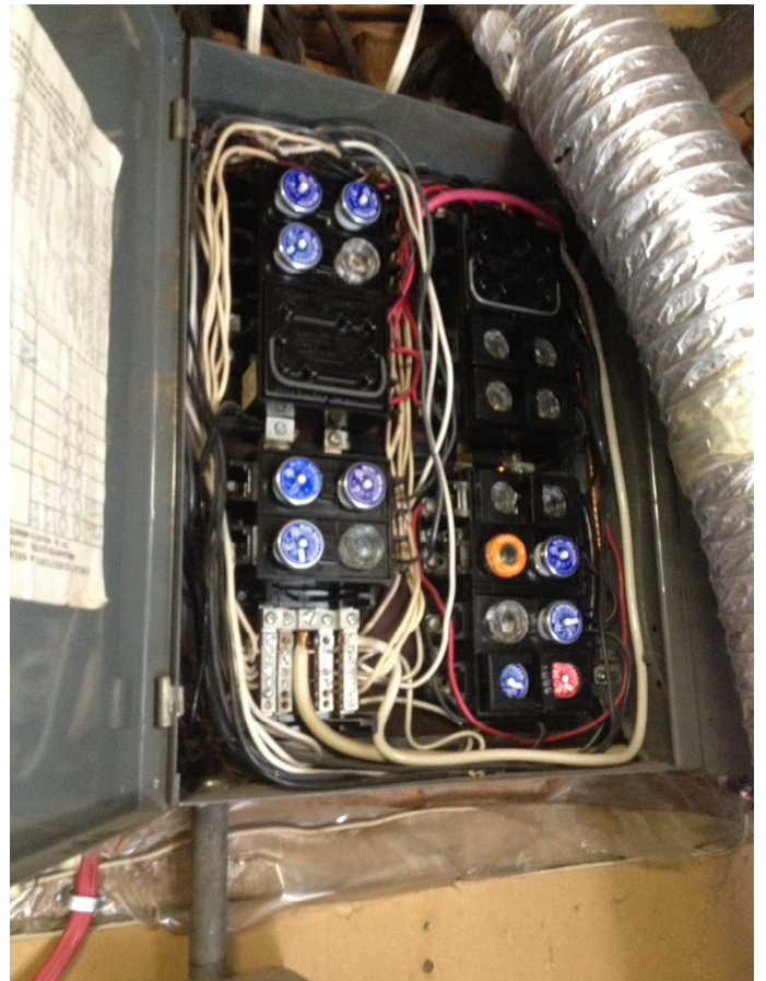
VERY dangerous - cover is missing. These wires are live!
